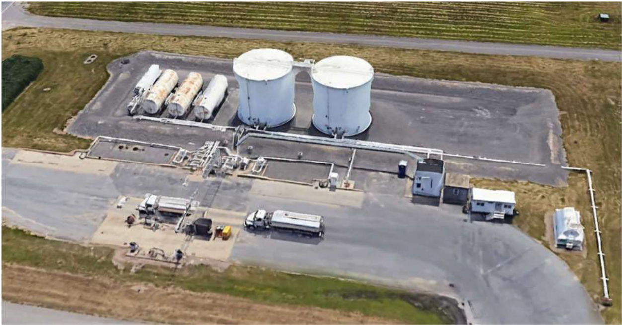
Figure 1 – Aerial View Site Work Location at Fuel Tank Farm
