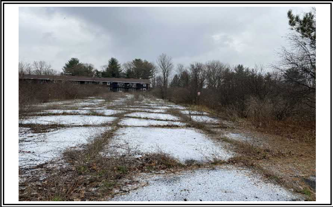
Photo 1 – View of paved road/path, facing east.
