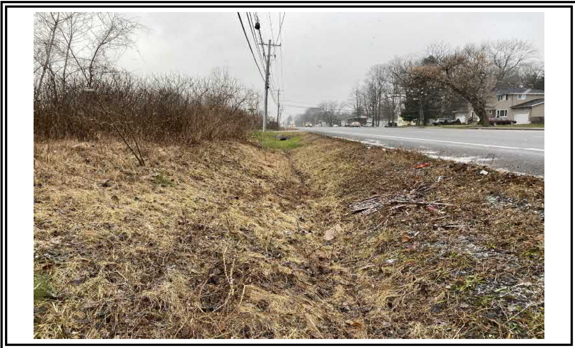
Photo 14 – View of upland roadside swale, facing west.
