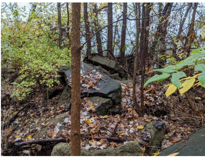
Photograph 3. Large concrete debris.
