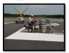
filling cracks, repainting the lines and replacing any runway lighting. The Airfield Maintenance division does this task twice a year for FAA specifications. They will go out again in September to repaint the center lines before the FAA inspection in October. While the runway was closed, all air traffic was using runway 15-33. The runway is now open and we would like to say "thank you" to the Airfield Maintenance division for all of your hard work!
